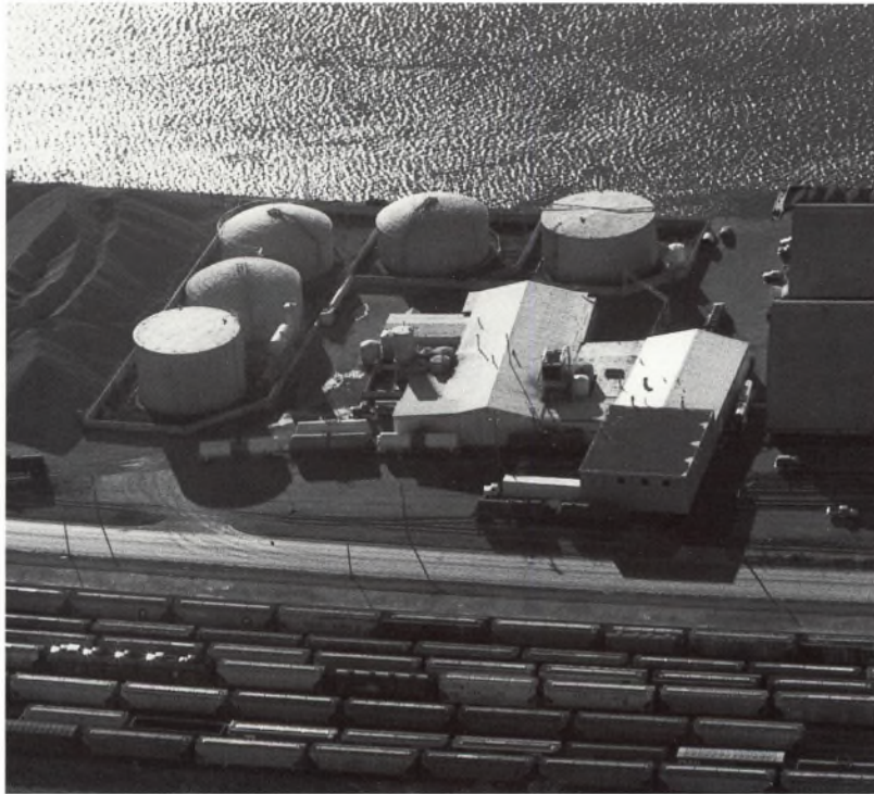
Terminal No. 1 on the Mississippi River in St. Paul.
